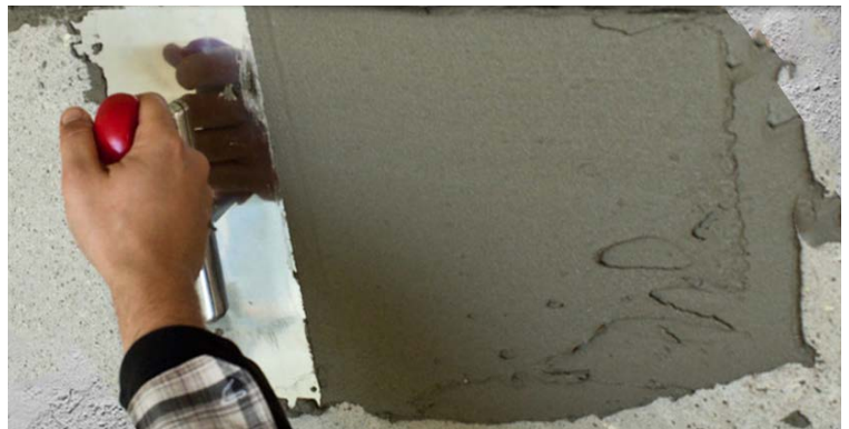
Fig. 2: Flat screed the adhesive.
