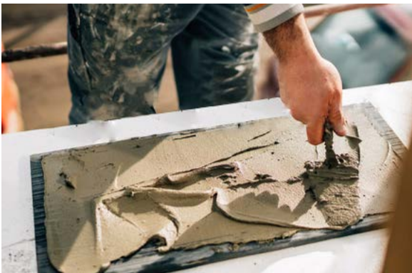
Fig. 3: generously back butter the stone.
